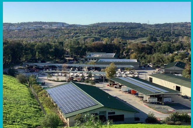
Figure 6 6. Solar Installation at Headquarters
