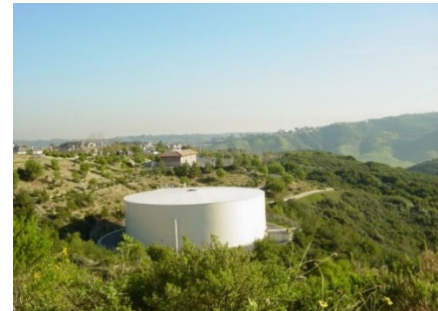
Aliso Viejo Recycled Water Reservoir
