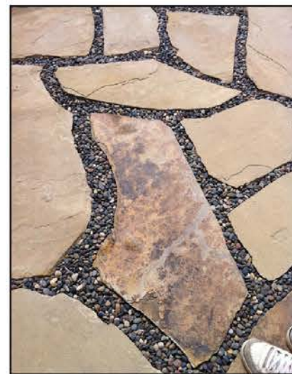
Permeable Paving (3" gaps for plants 1.5" gaps for birds eye gravel or dg fill)
