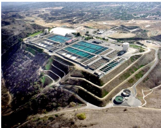
Diemer Filtration Plant
