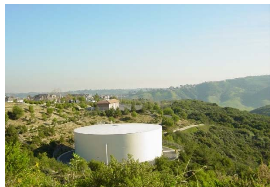
Aliso Viejo Recycled Water Reservoir
