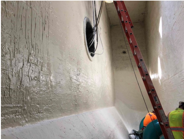
Inlet Piping into Wet Well While Under Bypass
