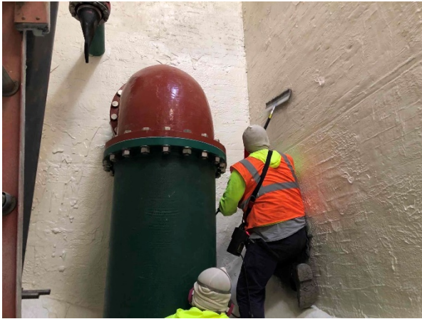
Testing of Coating on East Wall of Wet Well
