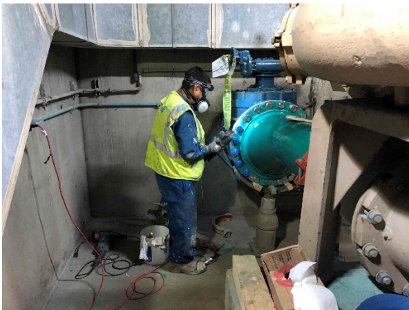
Dry Well Interior Piping Installation
