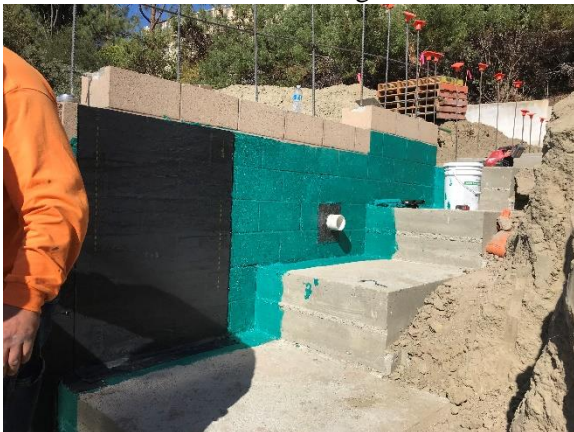
Water Proofing of Newly Built Wall
