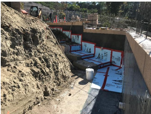
Preparations Prior to Site Backfill
