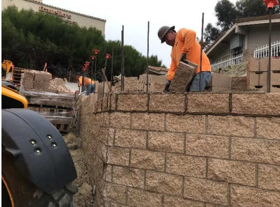
Construction of New Retaining Walls
