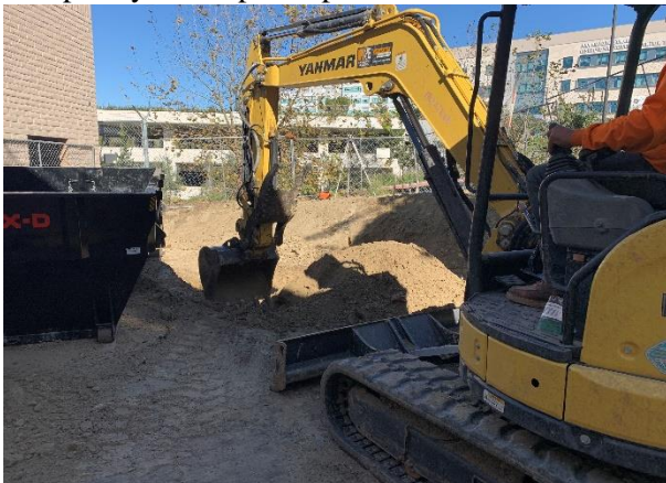
Grading of Slope for New Diesel Tank Location
