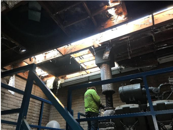
Removal of Existing Roof in Preparation for Removal of Equipment
