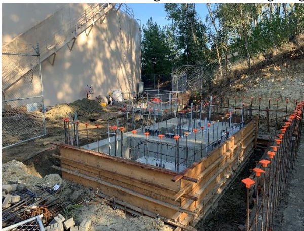
Aliso Hills Res. Building and Wall Foundation Prep
