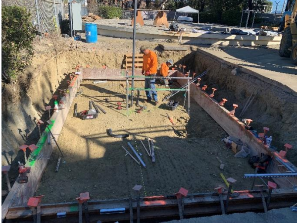
Forming Foundation and Conduit Installation at Aliso Summit Reservoir
