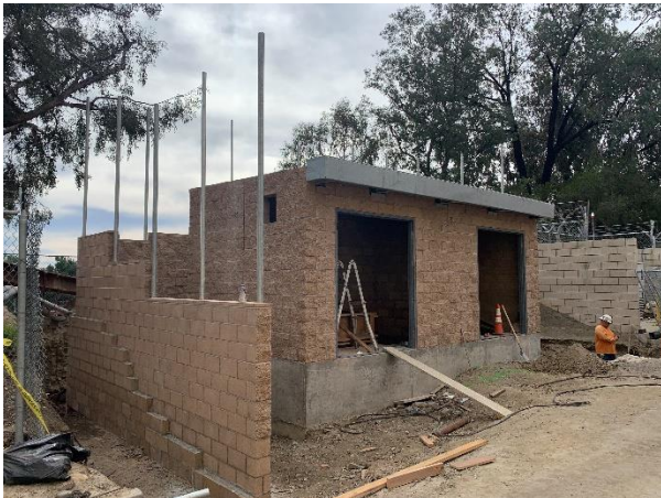
Bear Brand Res. Retaining Wall and Building Progress
