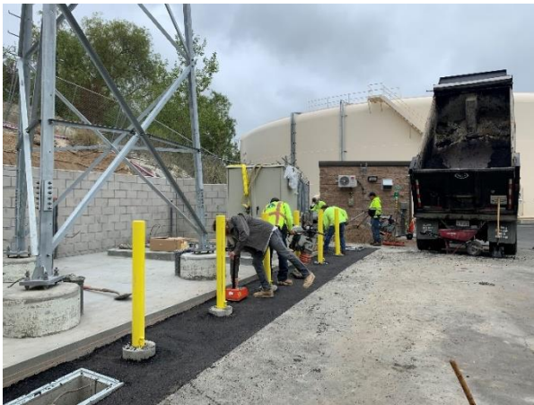
Installation of Final Paving
