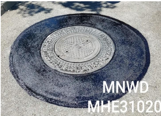
Completed Manhole Ring and Cover Rehabilitation
