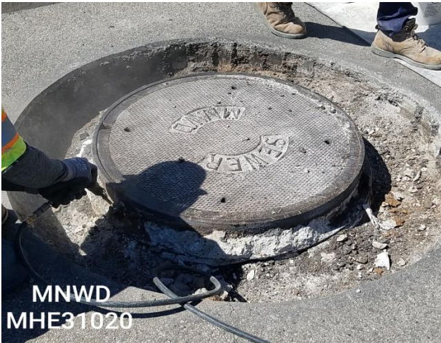
Manhole Ring and Cover Replacement
