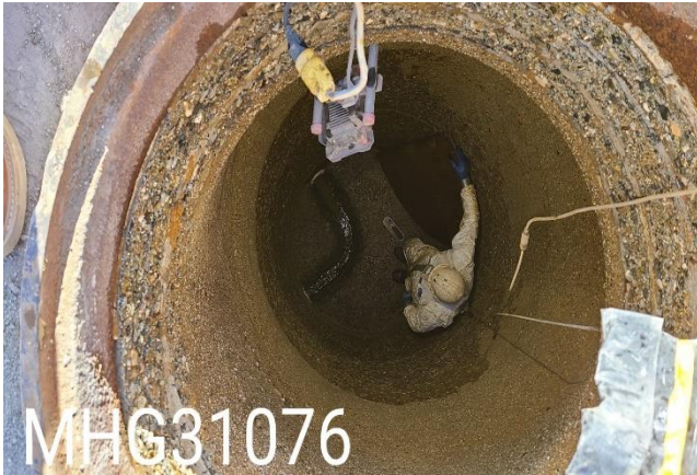
Manhole Rehabilitation Confined Space Entry
