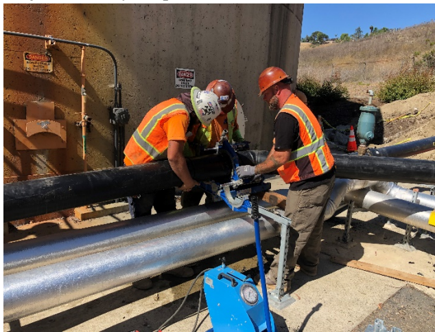
Crews Installation of Methane Gas Bypass Line
