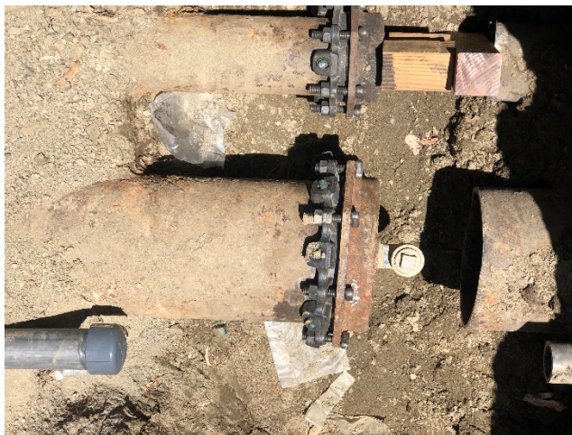
Excavation to Expose Methane Gas Line Connection
