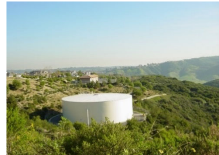
Aliso Viejo Recycled Water Reservoir
