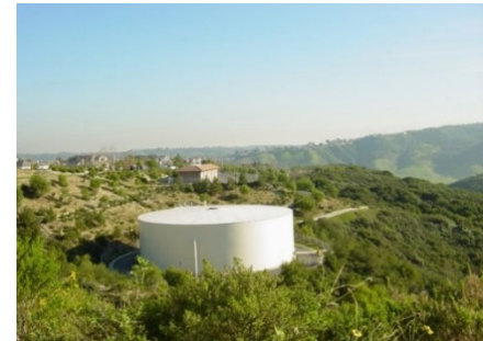
Aliso Viejo Recycled Water Reservoir
