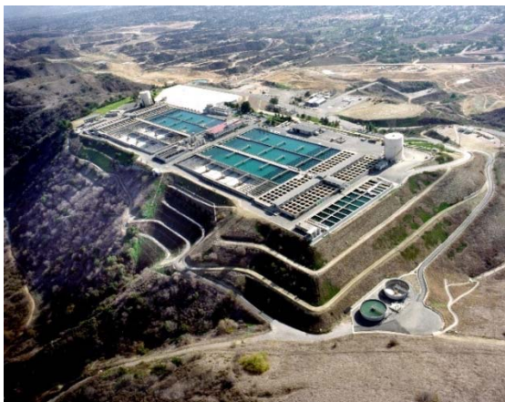
Diemer Filtration Plant
