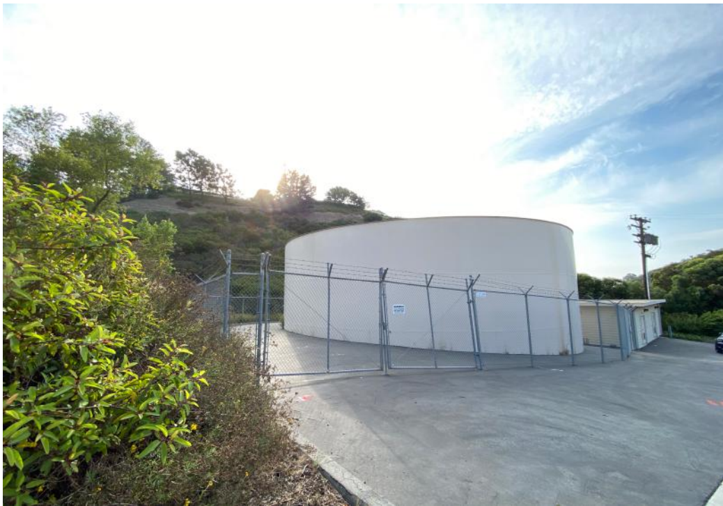
View from Pacific Island Drive looking at the existing Moulton Niguel Water District Facility and proposed Project site, looking southeast.
