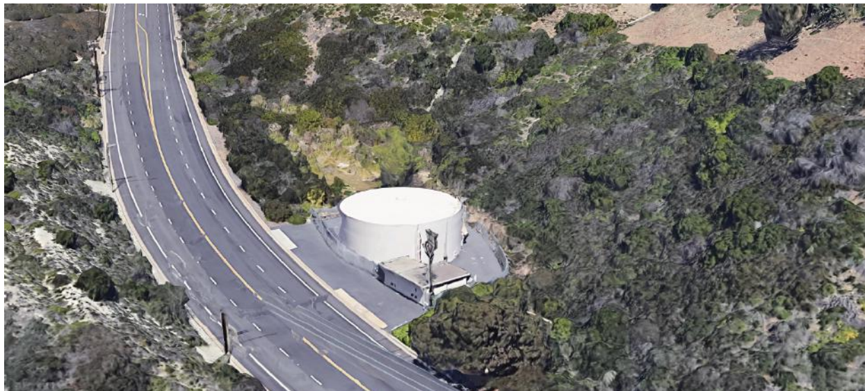
Figure 3 Pump Station Site (Before Proposed Project)
