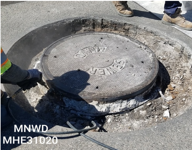
Manhole Ring and Cover Replacement
