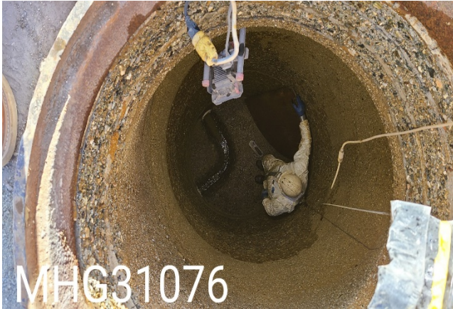
Manhole Rehabilitation Confined Space Entry
