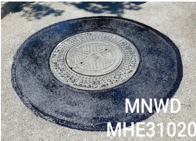
Completed Manhole Ring and Cover Rehabilitation
