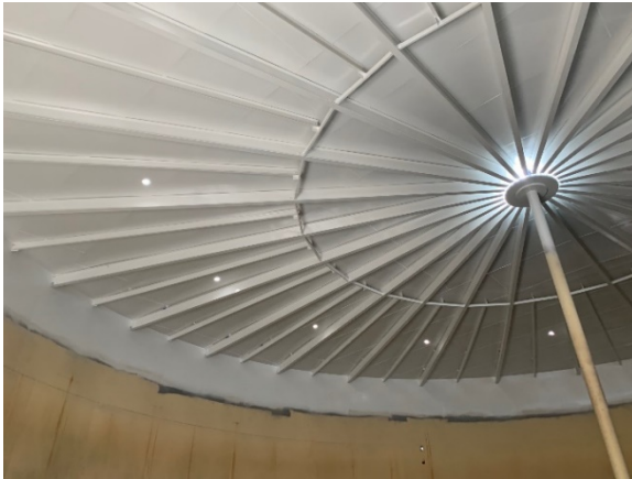
Newly Coated Interior Ceiling
