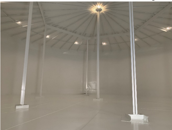
Completed Interior Coating Reservoir No. 1
