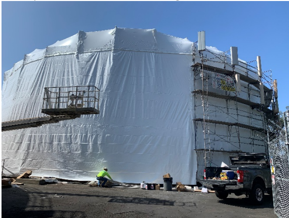
Containment Structure for Exterior Blasting
