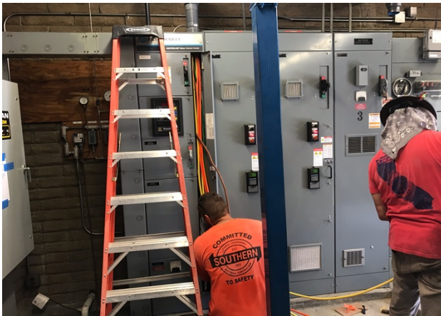
Installation of Switchgear Electrical at Big Niguel Pump Station
