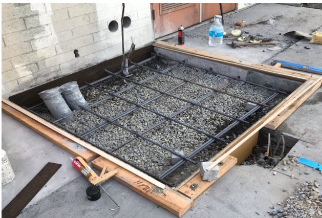
Preparation for New Equipment Concrete Pad
