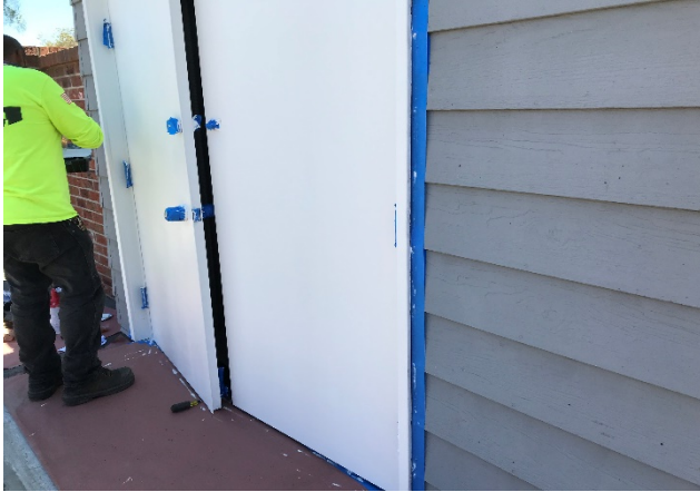
Newly Installed Doors at Existing Switchgear at Beacon Hill Pump Station
