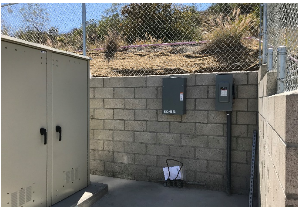
New Utility Main Breaker, ATS Box, and Electrical Enclosure
