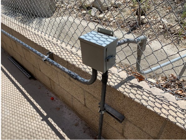
Newly Installed Communication Conduit
