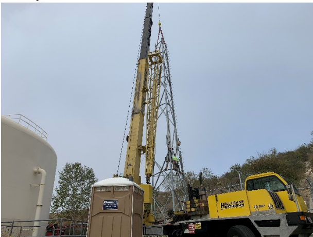
Installation of New Wireless Tower
