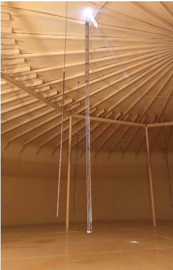
New Vortex Reservoir Mixing System
