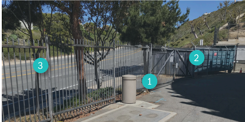
Photo 2: Inside PID II Reservoir Facility Looking North
