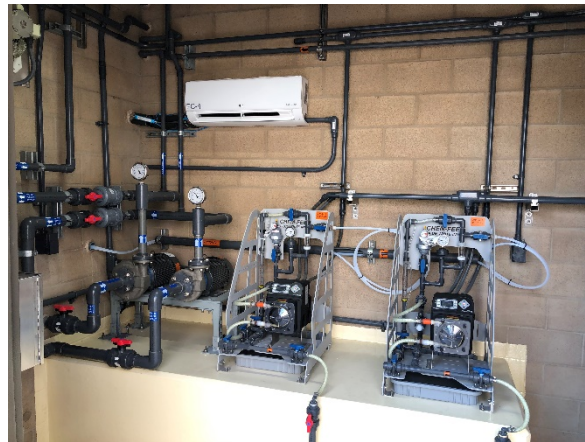
New Reservoir Mixing Pumps and Ammonia Metering Pumps
