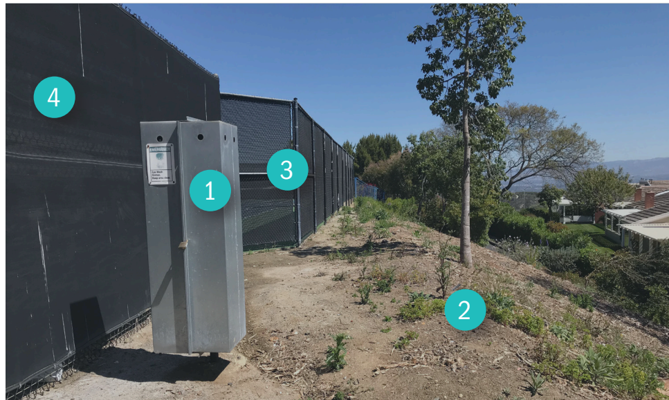
Photo 1: East of the Tennis Courts and RMS Building Looking North
