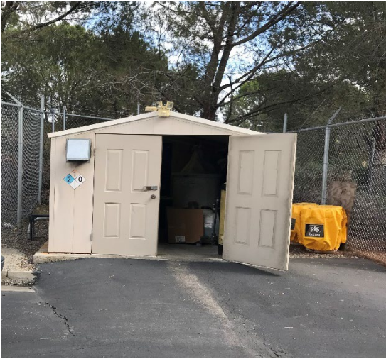
Existing OSG System Building to be Replaced
