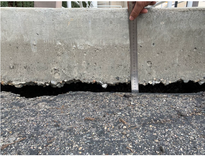
Ground Subsidence at Stair Landing
