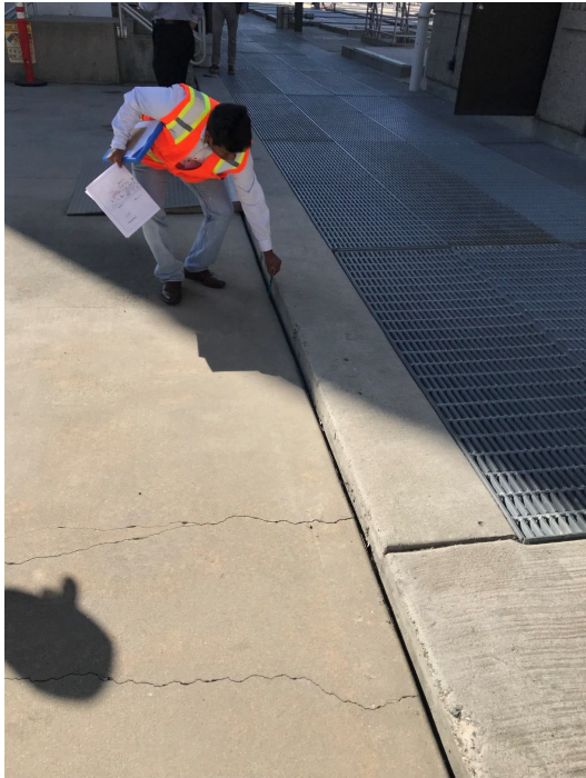
Concrete Settlement and Distress at Pipe Tunnel
