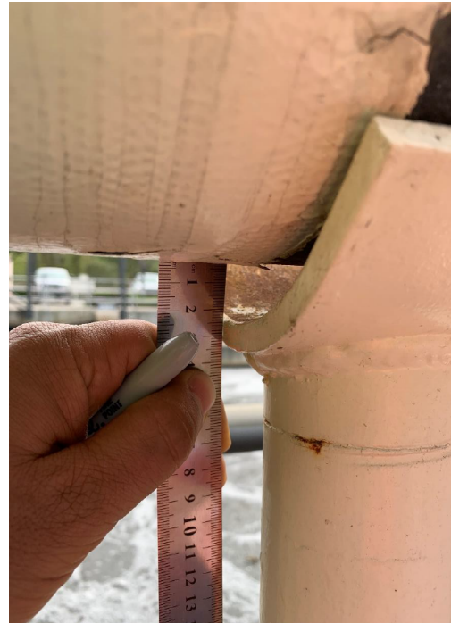
Settlement at Pipe Support
