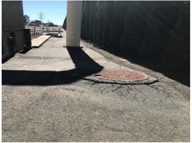
Pavement Distress at Manhole and Pipe Riser
