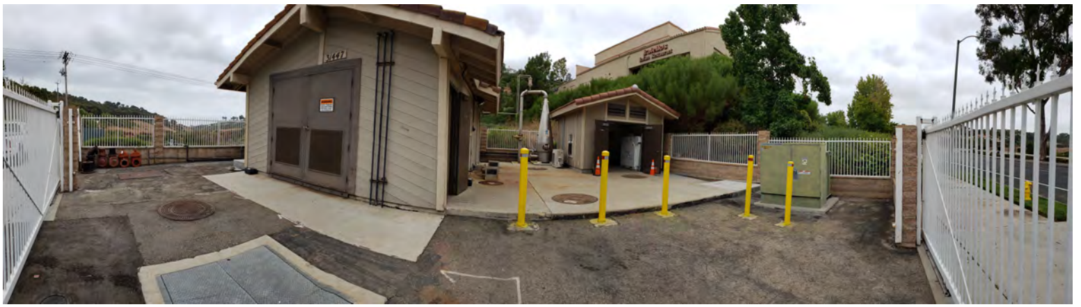
Upper Salada Lift Station (panoramic)
