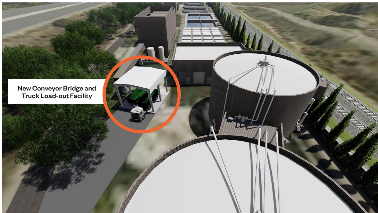
Figure 11. 3-D Modeling with constructing a new conveyor bridge and truck loadout facility for easy access and larger bins.
