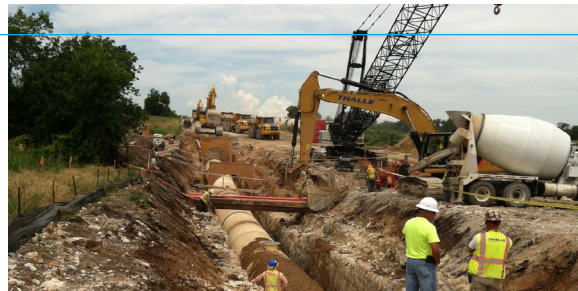
Romeo has successfully served as construction inspector for the Brackish Water Desalinization project and the Central Water Integration Project. Both involve water treatment plants, tanks, pump stations and 55,000 feet of pipelines.
