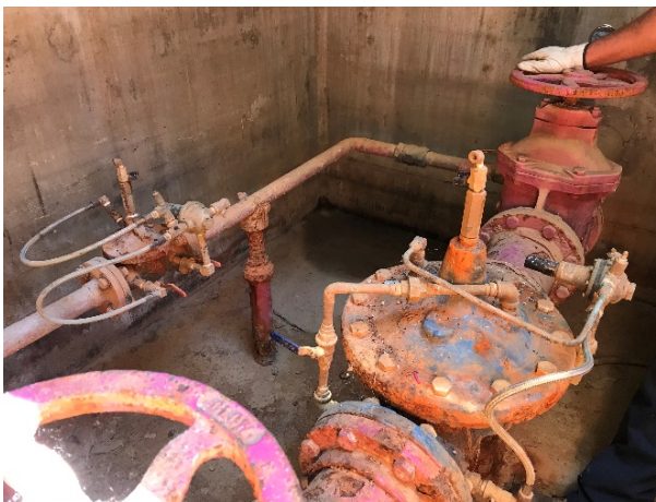
Valves and Piping to be Replaced at Wood Canyon
