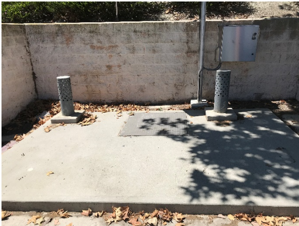
Wood Canyon Pressure Reducing Station
