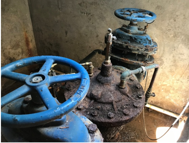
Valves and Piping to be Replaced at Canyon Wren
