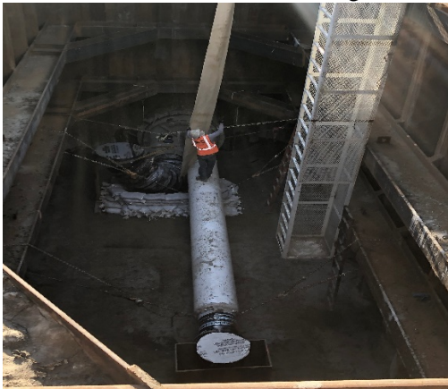
Placement of Thrust Blocks for New Pipelines
