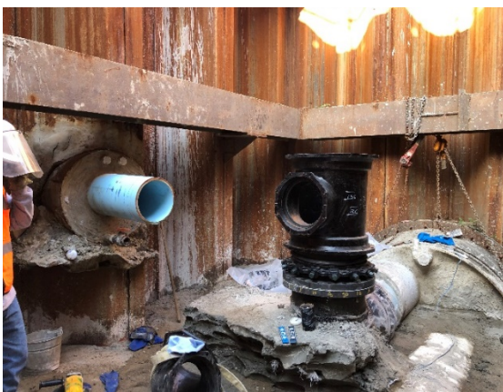
Installation of New 20-inch x 12-inch Potable Water Connection
