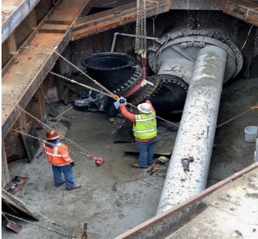
Installation of 30-inch DIP Fittings
