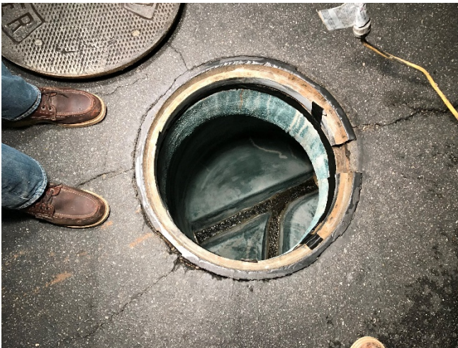
Manhole Channel Repair Example
