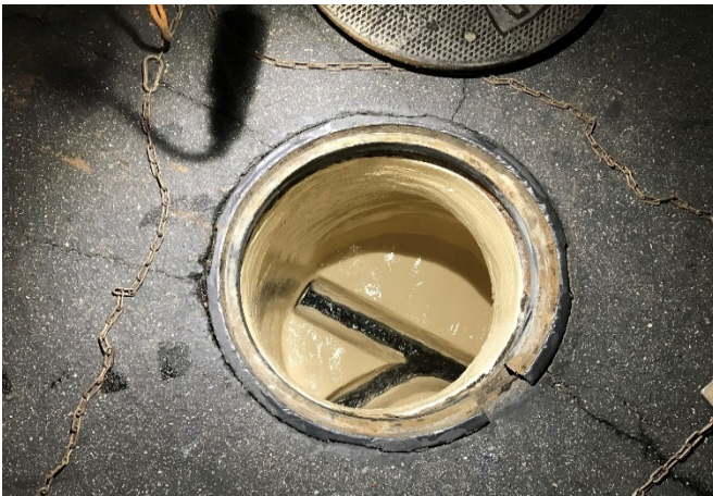
Manhole Rehabilitation Example
