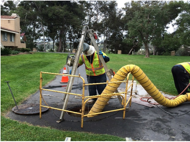
Manhole Rehabilitation Confined Space Entry
