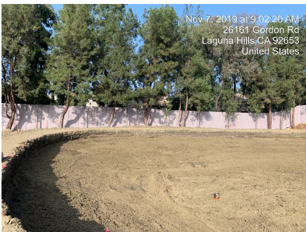
Newly Installed Sound Blankets
