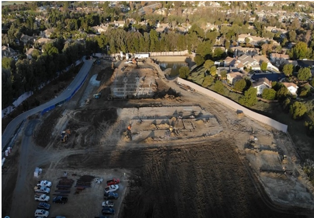
Aerial View of Demolition and Site Improvements
