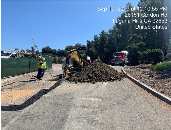
Installation of Temporary Sewer
