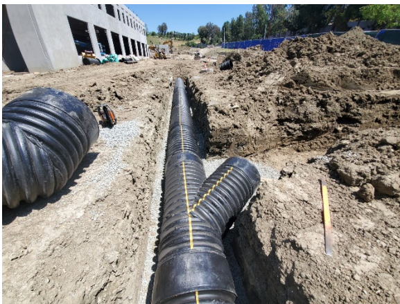
On-site Storm Drain Installation
