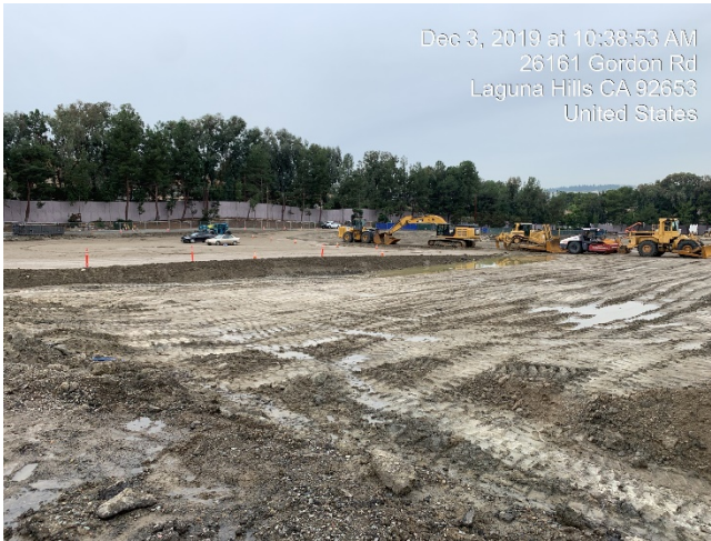
Grading and Site Reconfiguration
