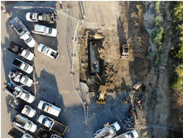
Removal of Existing Fuel Storage Tank
