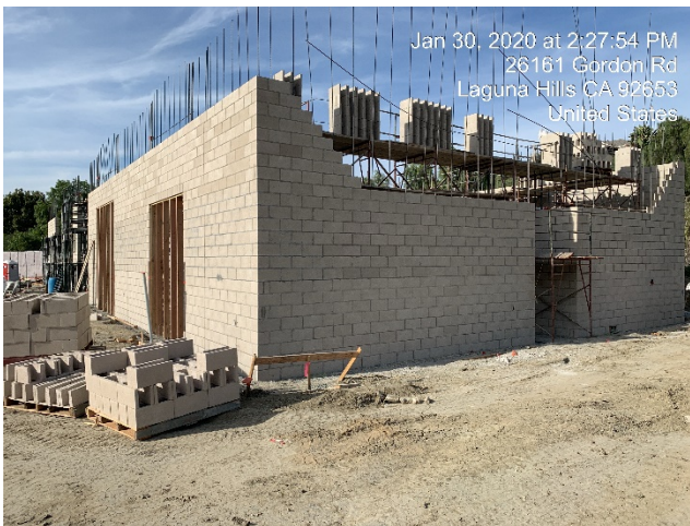
Progress of New Fleet Services Building
