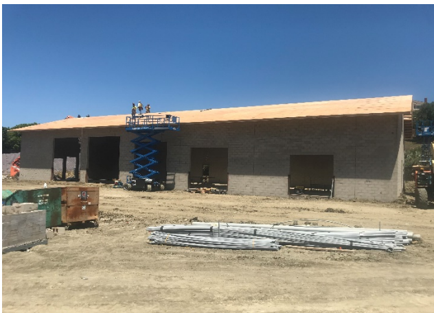
Current Construction of New Fleet Building
