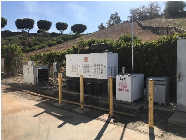
Existing Emergency Generator
