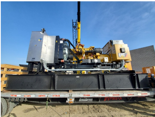
Arrival of New Generator
