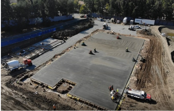
Aerial View of Newly Poured Slab
