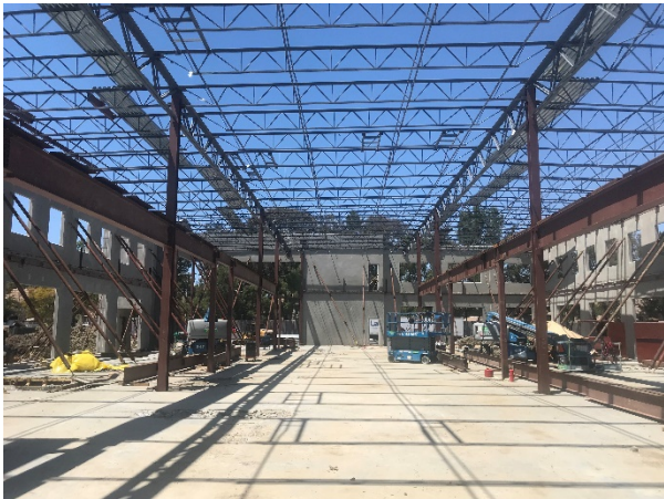
Interior Construction of Administration Building
