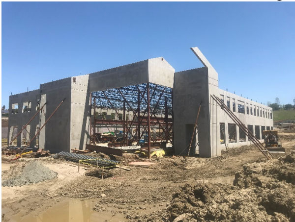
Exterior Construction of Administration Building
