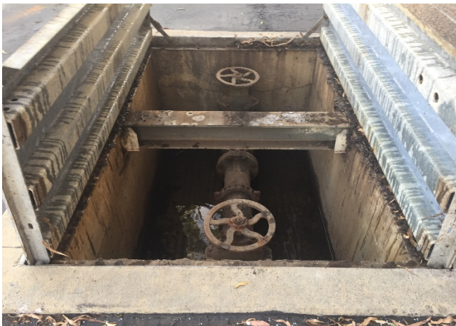
Existing Valve Vault to be Replaced
