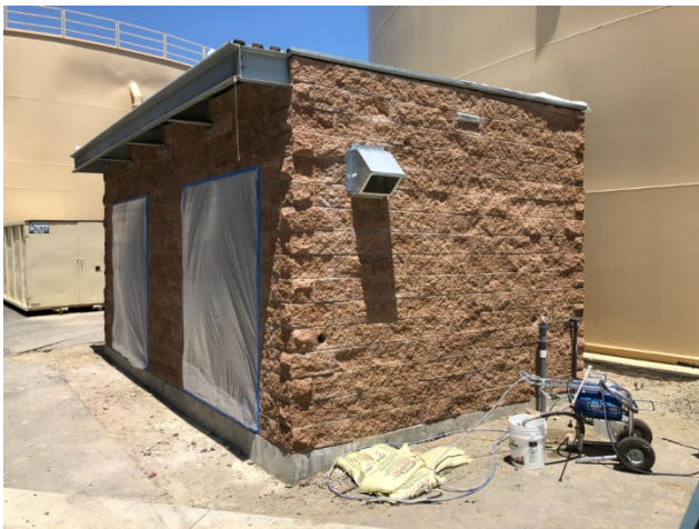
New RMS Building at Crown Valley Reservoir
