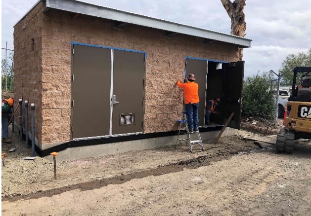
Building Construction Continues at Marguerite Reservoir
