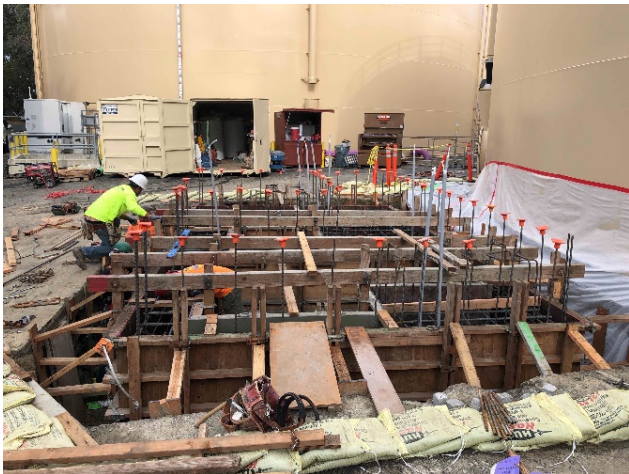
Building Foundation Prep at Crown Valley Reservoir
