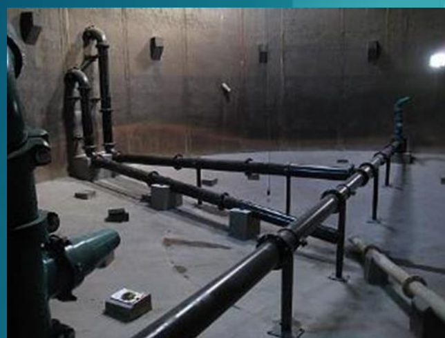
External Pumped Nozzle Digester Mixing
