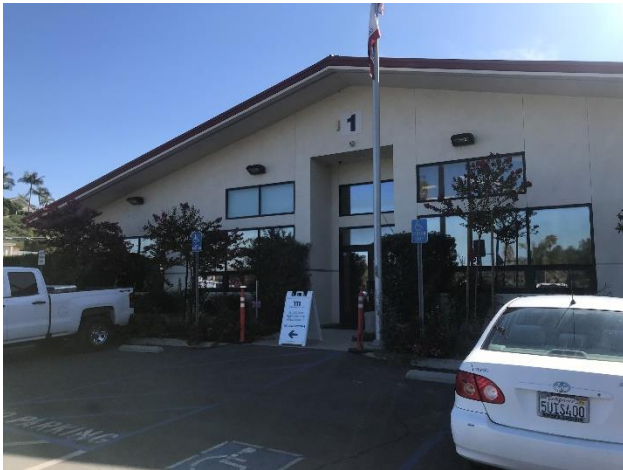
Existing Field Operations Building to be Reconfigured to New Warehouse
