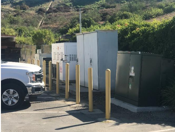
Existing Utilities to be Upgraded
