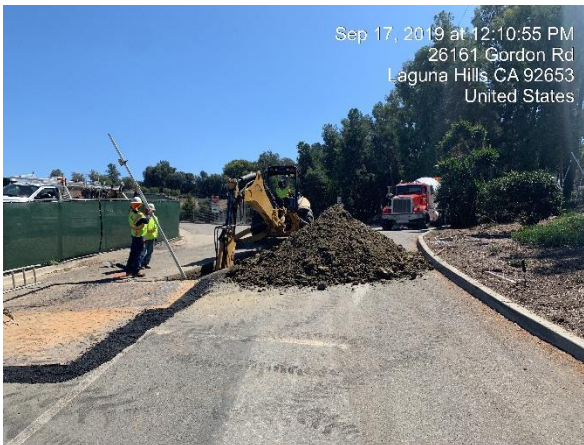
Installation of Temporary Sewer
