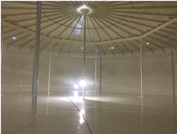
Completed Interior Coating
