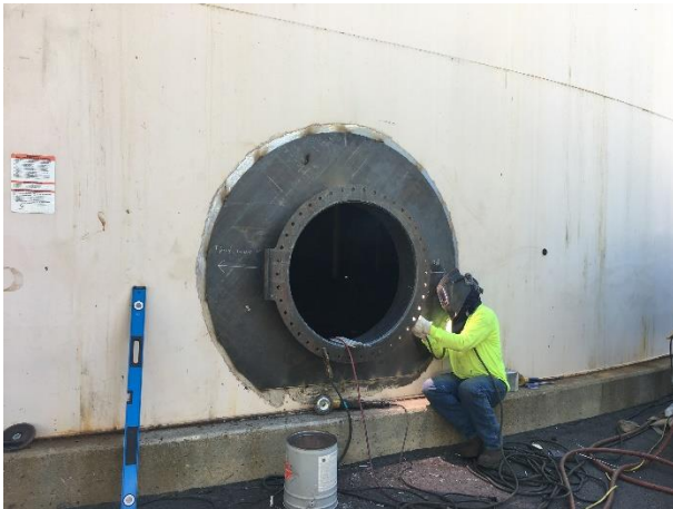
New Manway Installation
