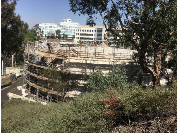
Preparation for Exterior Coating
