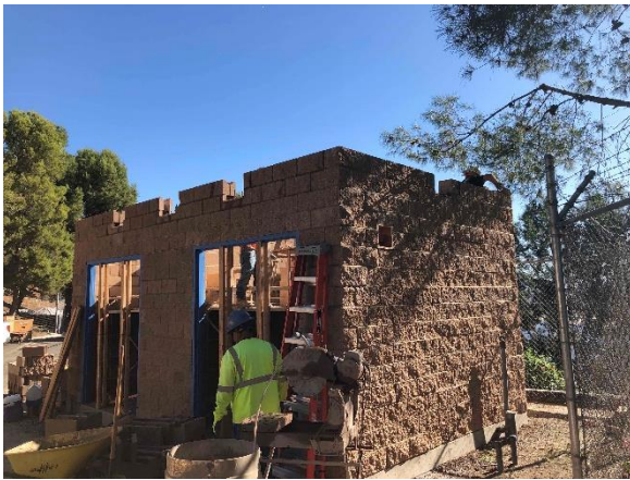
New RMS Building at Pacific Park Reservoir
