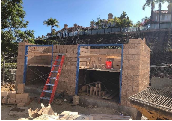
New RMS Building at Highlands Reservoir
