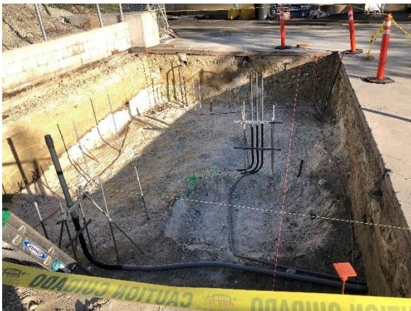
Preparation of Building Foundation at Moulton Peak Reservoir
