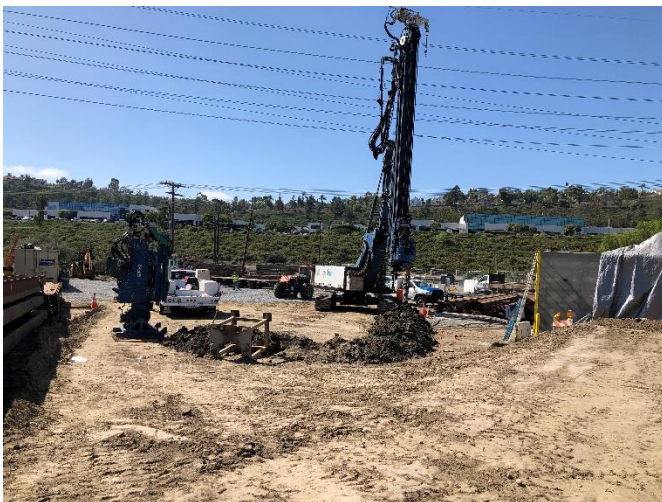
Excavation Work for Launch Pit
