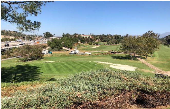
Crews Begin Preparing Receiving Pit Location
