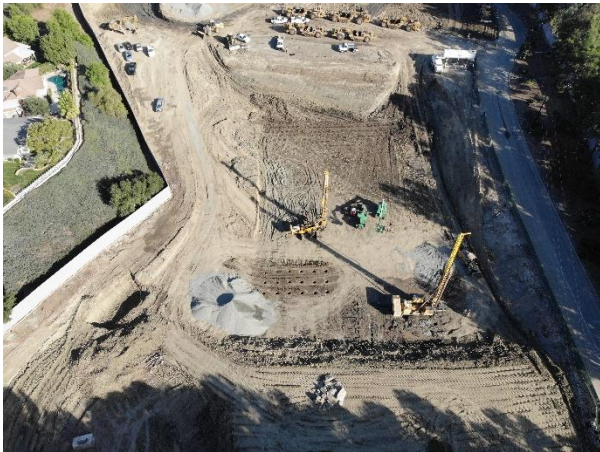
Current Site of Field Maintenance Facility
