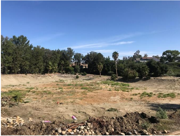
Original Site of Field Maintenance Facility
