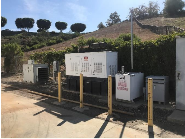
Existing Emergency Generator
