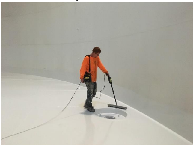
Interior Coating Spark Test Being Performed
