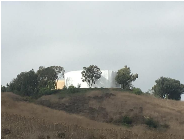
Bear Brand Reservoir Exterior Containment Prior to Coating
