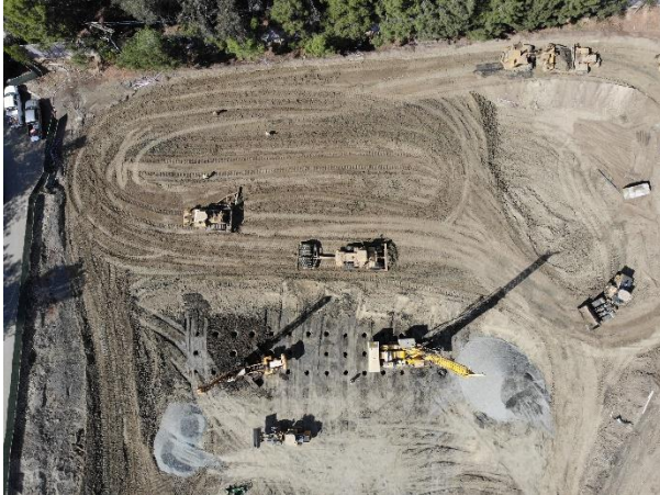
Current Site of Administration Facility
