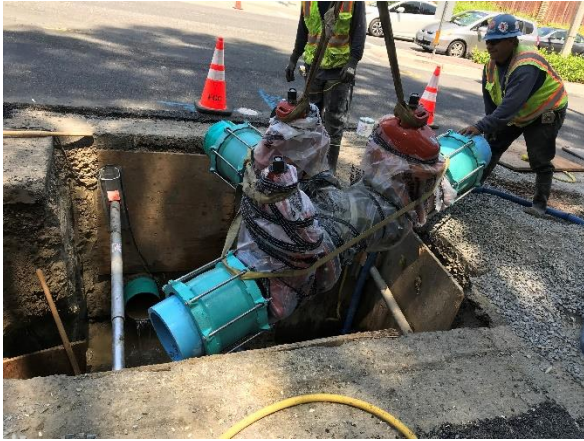
Installation of New Valves and Tee at Spadra and La Paz in Mission Viejo
