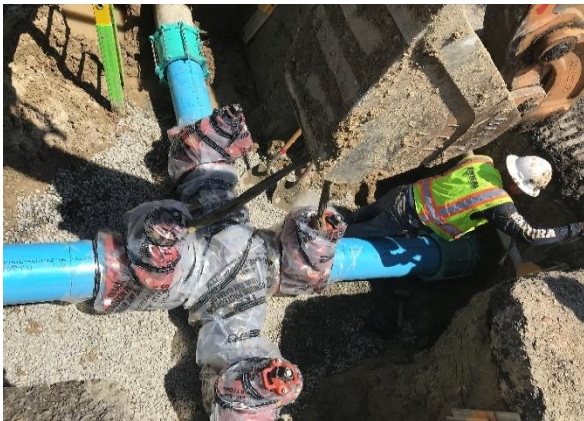
Valve Replacement at Trabuco and Los Alisos in Mission Viejo
