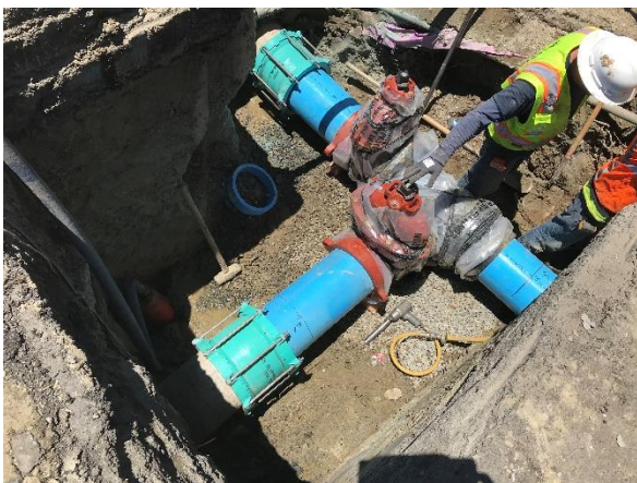
New Valves at Marina Hills and Golden Lantern in Laguna Niguel
