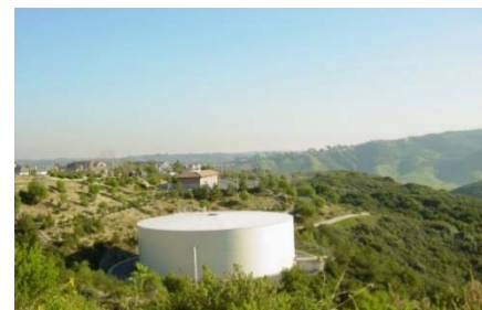
Aliso Viejo Recycled Water Reservoir
