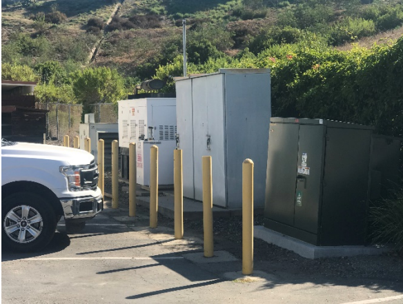
Existing Utilities to be Upgraded
