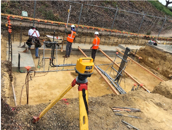
Excavation for New RMS Building at Highlands Reservoir
