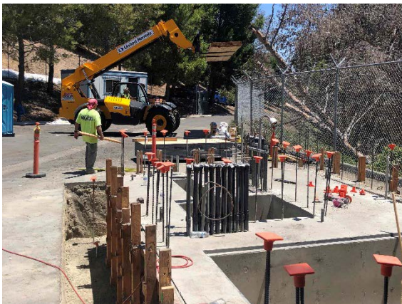
Newly Placed Building Foundation at Pacific Park Reservoir
