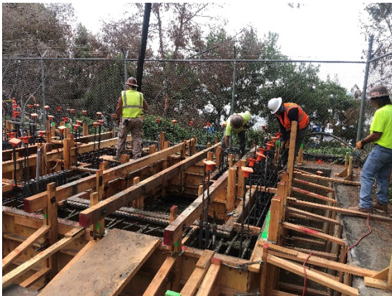
Framing for Foundation Placement at Pacific Park Reservoir
